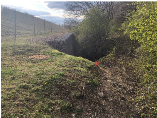
Figure 3: Gabion wall with red flag identifying the land registry boundary line
