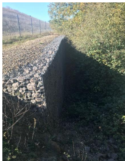
Figure 4: Gabion wall at point 2
