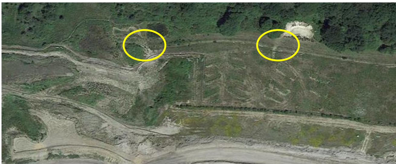
Figure 6: Satellite Image of Northern Boundary Run-off Issues
